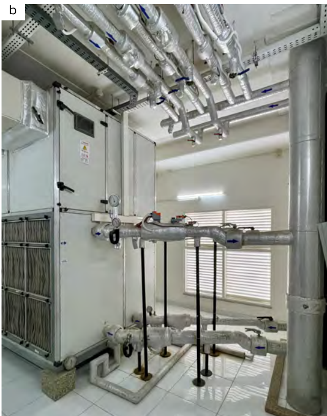
Figure 5.3: (a) Smooth and obtuse angle bends in chilled water piping, (b) Piping and ducting at AHU with minimum bends
