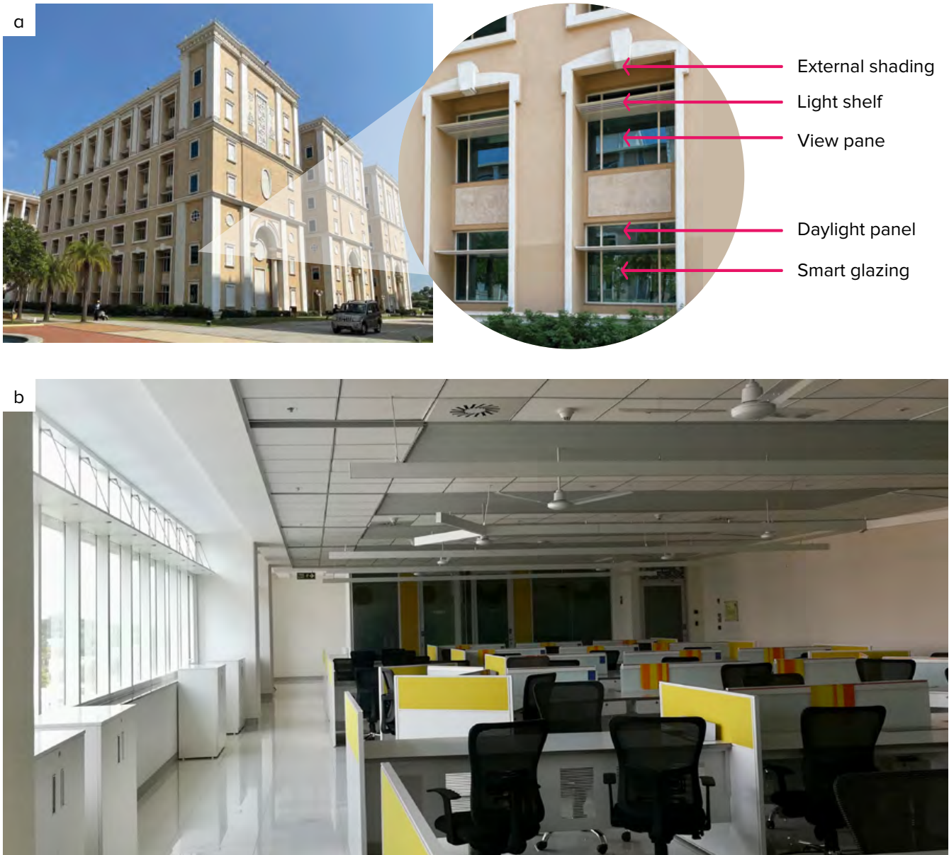
Figure 5.1: (a) Components of façade design, (b) Daylit interiors due to daylight panels and light shelves
